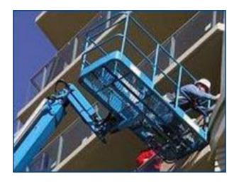
All operators must demonstrate that they understand how to use the lift and must be retrained if they do not demonstrate the skill or understanding needed for safe operating procedures.
