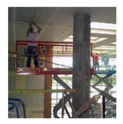
All aerial lifts require fall protection. Guardrails and buckets provide some fall protection but due to the "catapulting" characteristics of lifts it is necessary to have additional fall protection.
