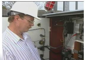
6. Verification of isolation. Before starting work on the machine that has been locked out or tagged out, the authorized employee should verify that the isolation of the machine or equipment has been achieved.
