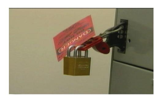
Lockout/Tagout is required to ensure that, before any employee performs any servicing or maintenance on a machine or equipment where the unexpected energizing, start-up or release of stored energy could occur and cause injury, the machine or equipment must be isolated from the energy source and rendered inoperative.
