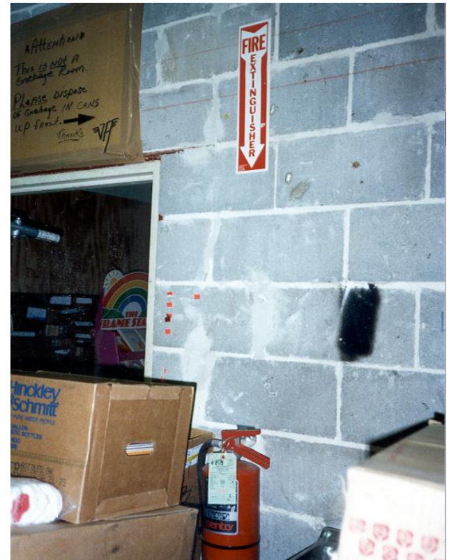
Blocked extinguisher
